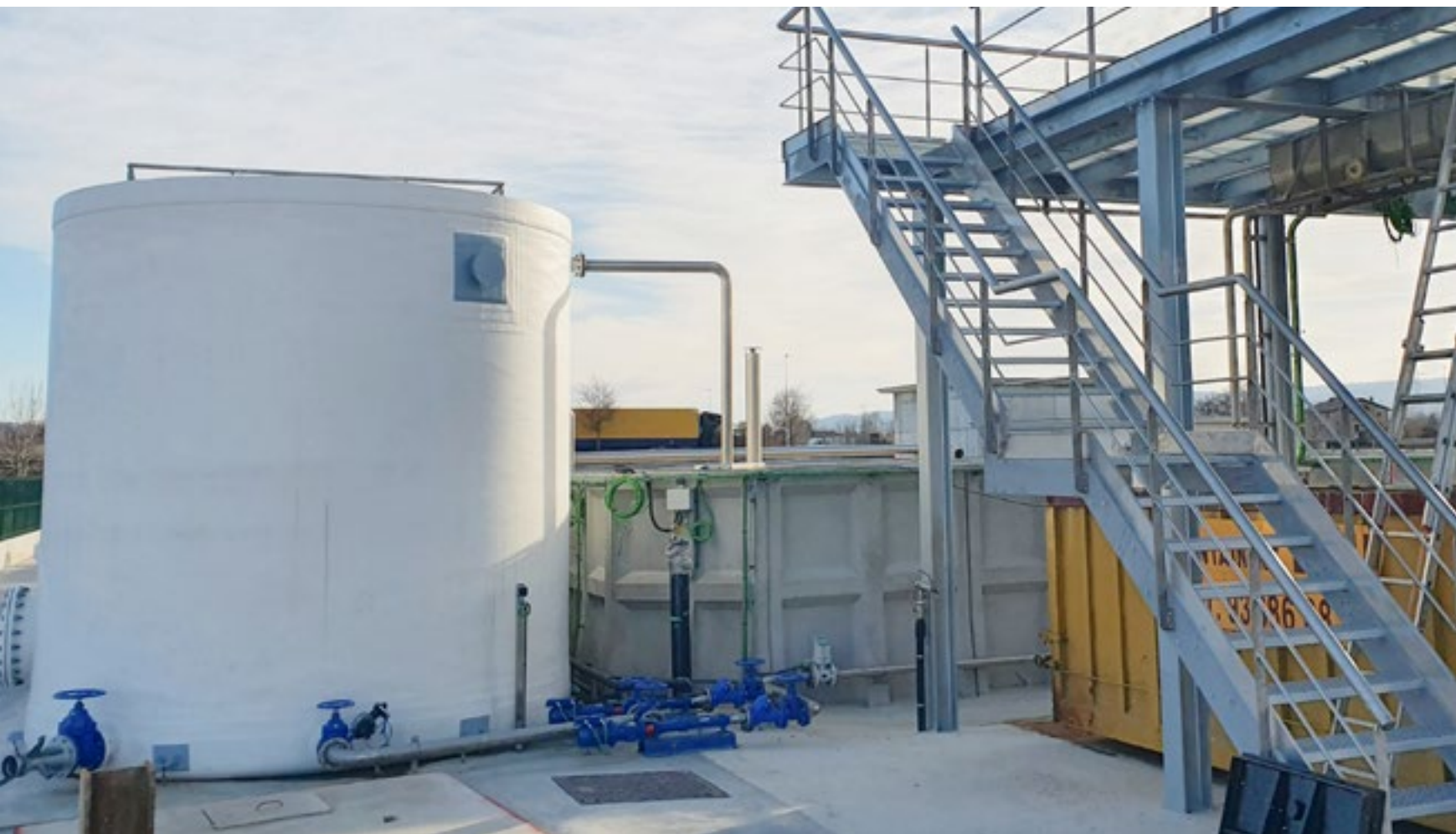
Sludge treatment tank and dewatering system
