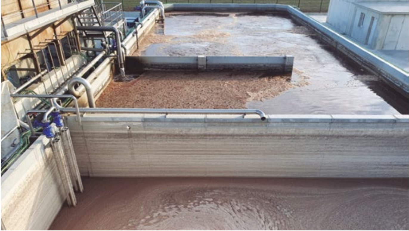
Aerobic homogenization tanks at a biological wastewater treatment plant using a membrane ultrafiltration system
