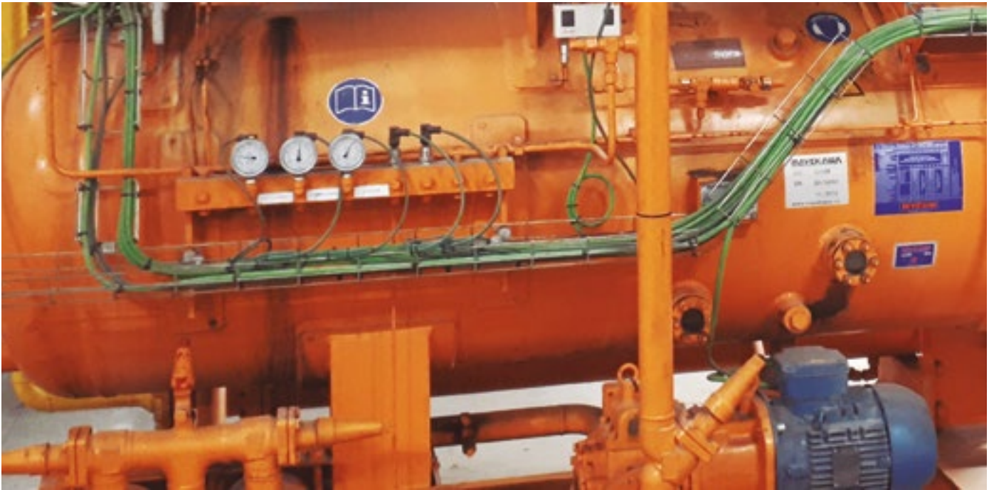
Auxiliary compressor equipment
