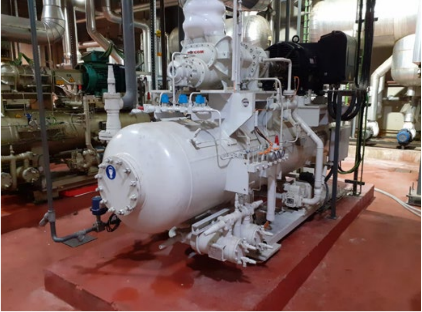
Refrigeration compressor
